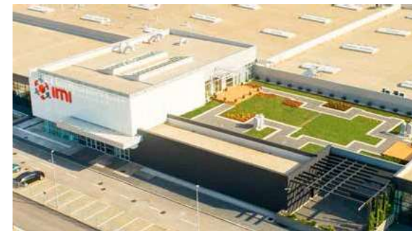
IMI Serbia with over 50,213 sqm of factory space is using 100% green energy.
